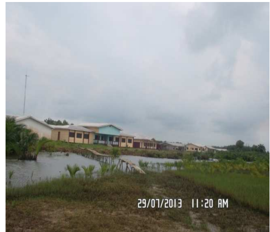
Buildings hosting D.O's Office and most Ministerial departments at Idabato II
